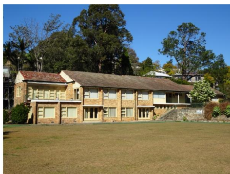
Former bowling club building
